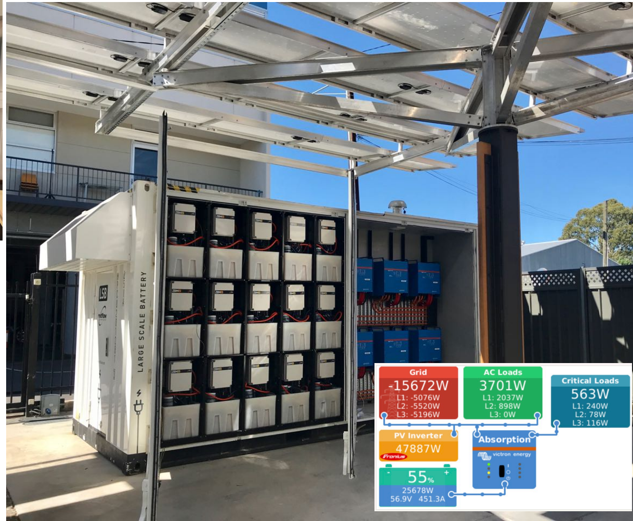
450kWh Battery / 100kWp Solar for solar self-consumption & backup
